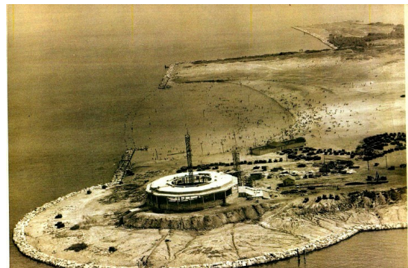
1929 aerial, showing construction of Adler planetarium, the filling operations at 12 th Street Beach.
