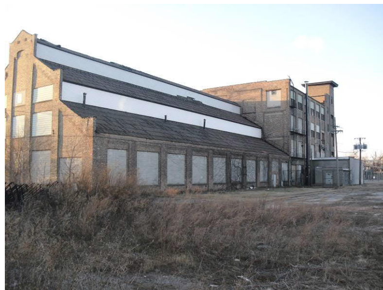
Photo 12: View of the north adjoining property facing northwest.
