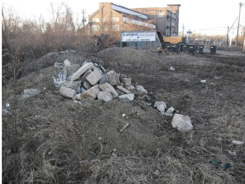
Photo 11: View of the dirt, gravel, concrete, shredded plastic, and dumpsters located on the northeast portion of the site.
