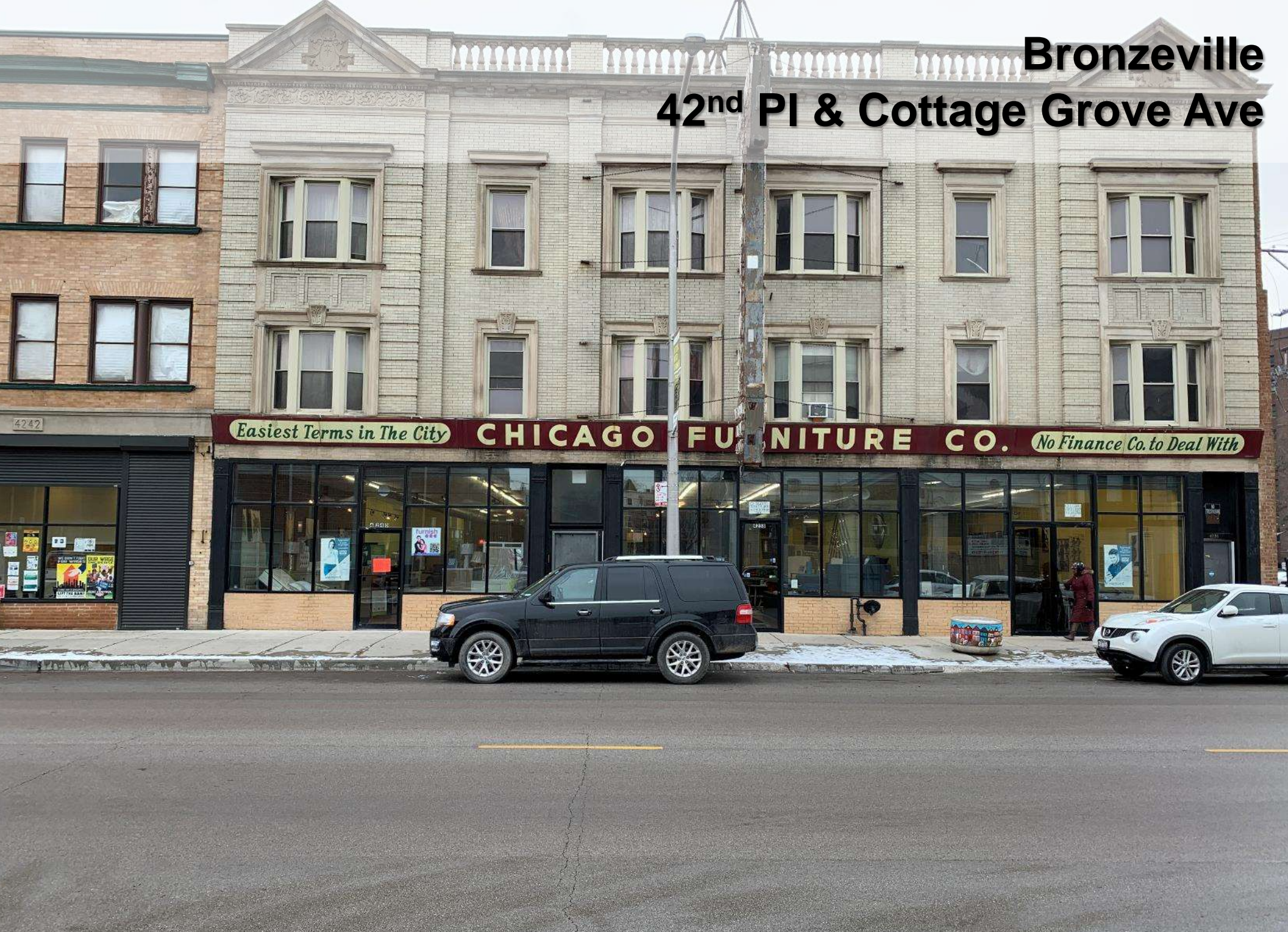
Existing Furniture Store
