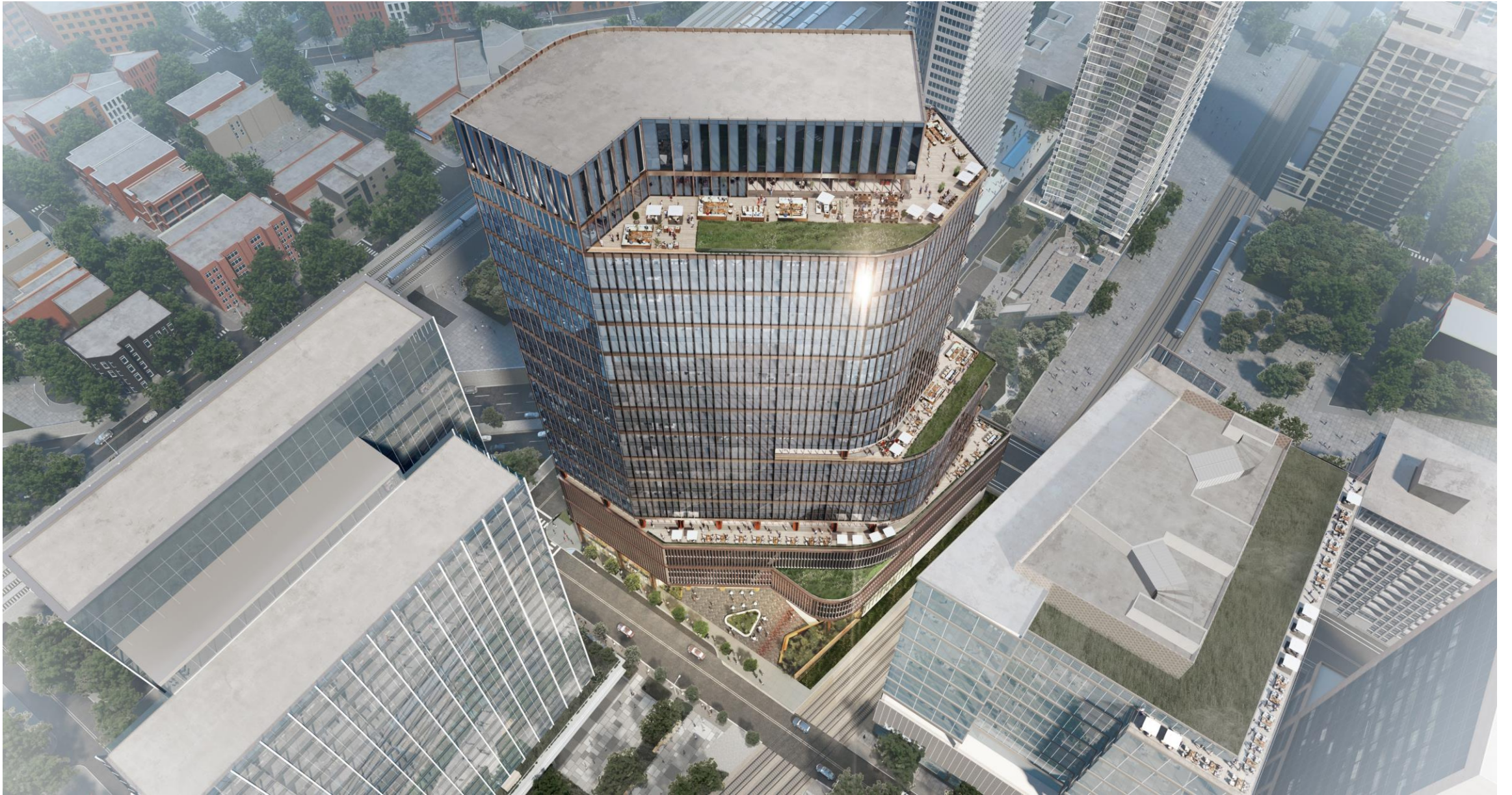
BUILDING OVERALL IMAGE (From SouthWest)
