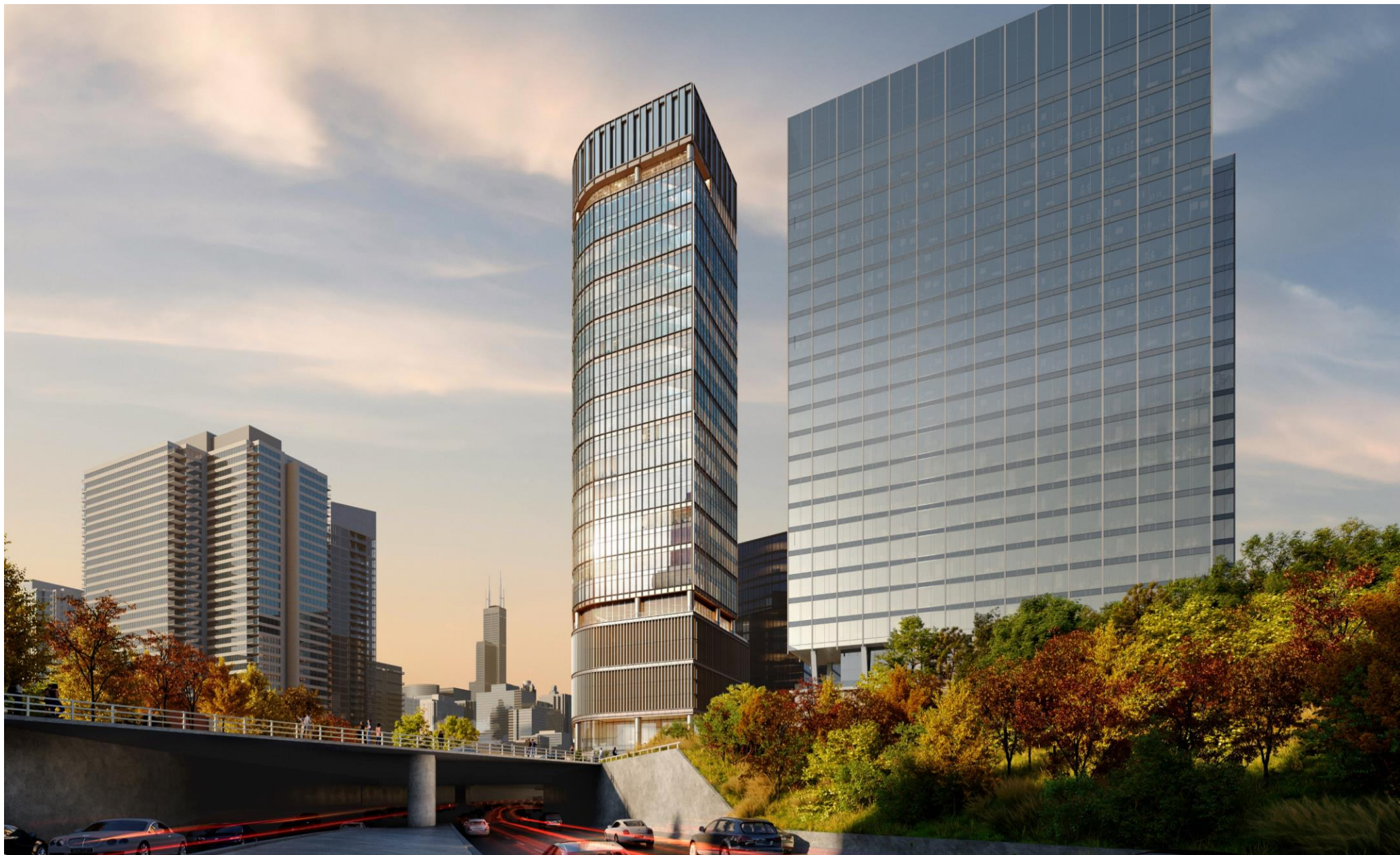
BUILDING OVERALL IMAGE (From NorthWest along I-90/94)
