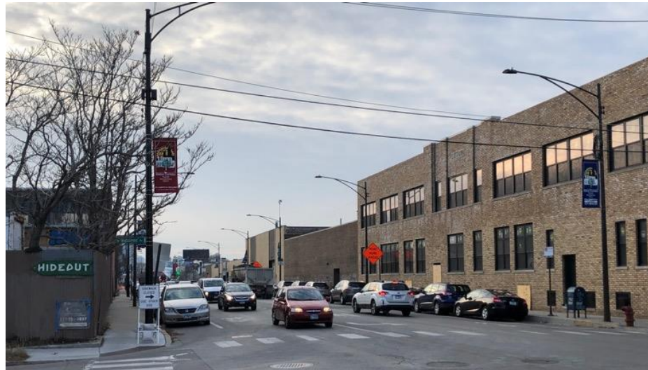
Elston Avenue, looking SW from West Wabansia Avenue. Project building is on the right.
