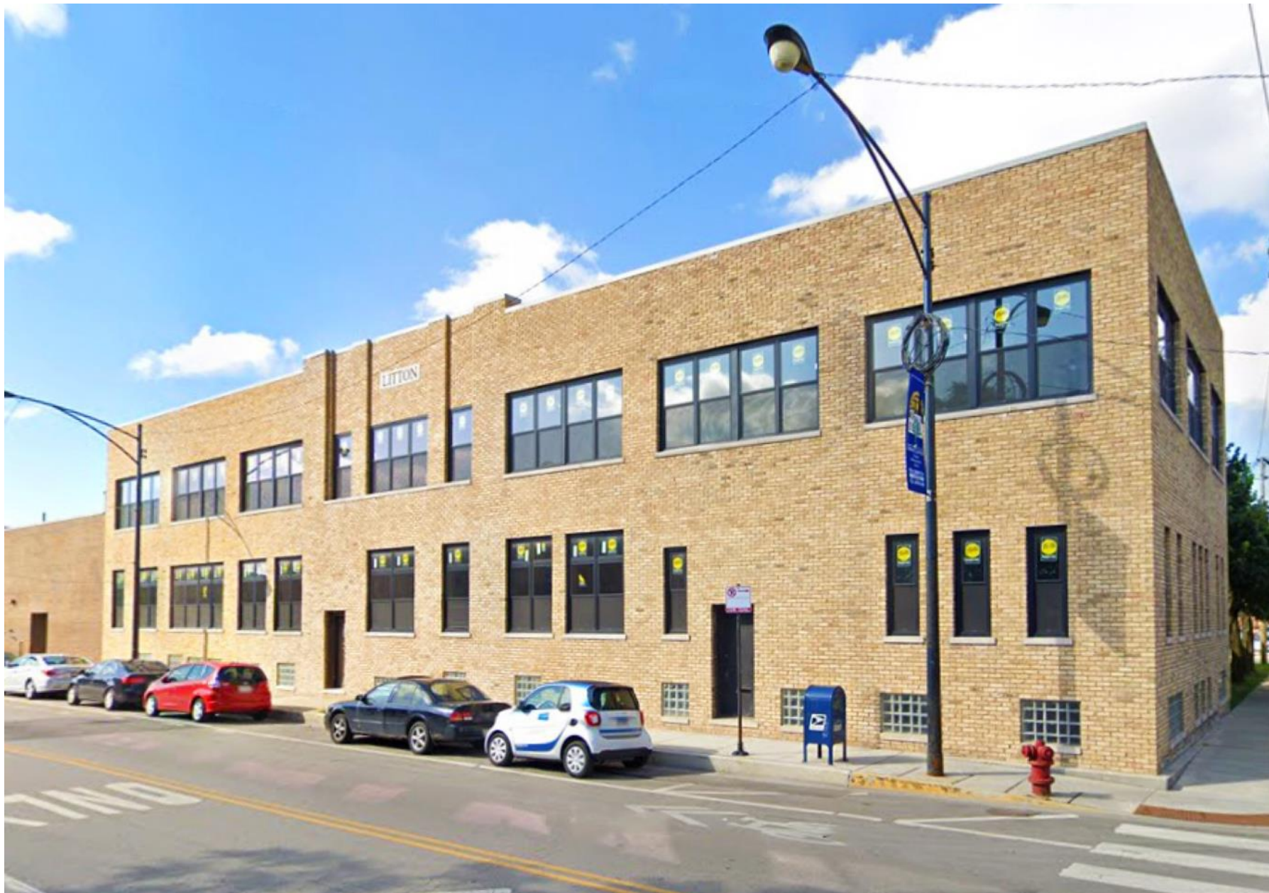
EXISTING BUILDING – ELSTON AVENUE
