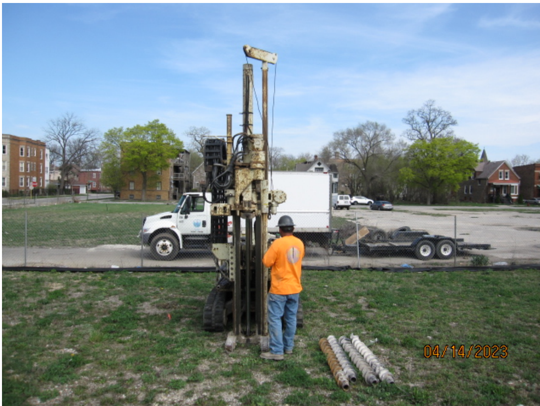
Photo 20: Drilling activities at B-6a (typical).
