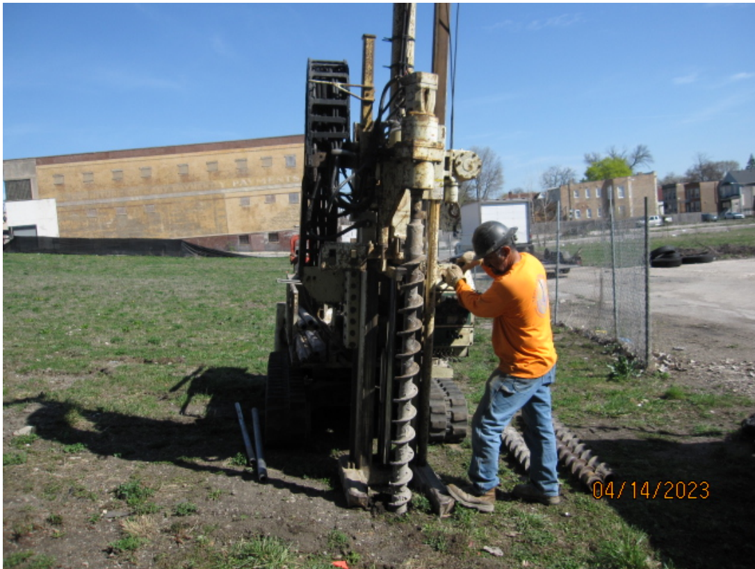
Photo 17: Drilling activities at B-12a (typical).
