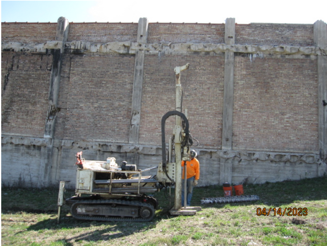
Photo 19: Drilling activities at B-11a (typical).
