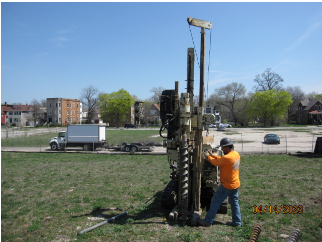
Photo 18: Drilling activities at B-8a (typical).
