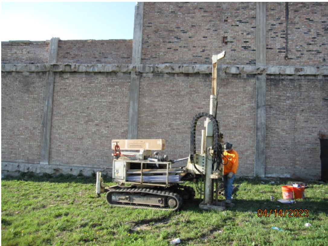
Photo 16: Drilling activities at B-10a (typical).
