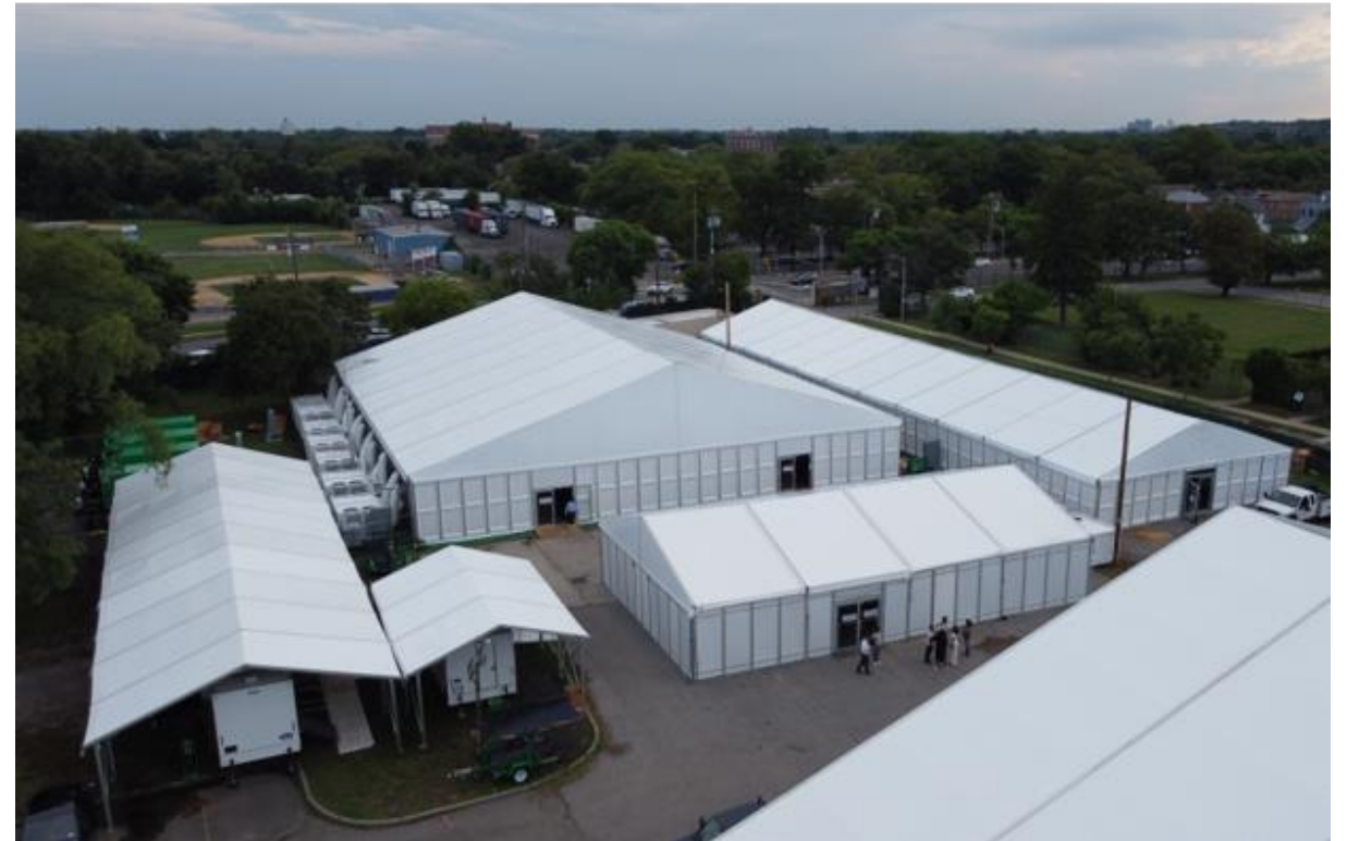
GardaWorld Federal Services Shelter in New York City
