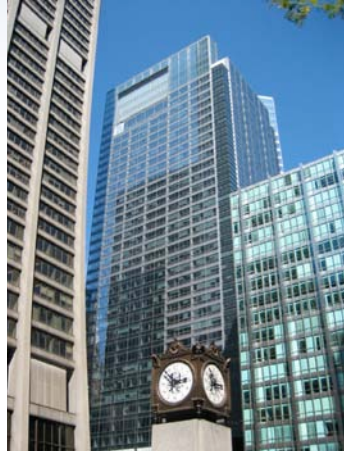
Image 1-2: Infill sites in the Central Loop are being developed as Class A office space.
