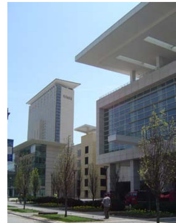
Image 1-16: Recent expansion of McCormick Place will drive the need for improved facilities for business visitors.
