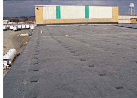
Billowing of roof membrane can cause air intrusion from the interior into roof assembly.
