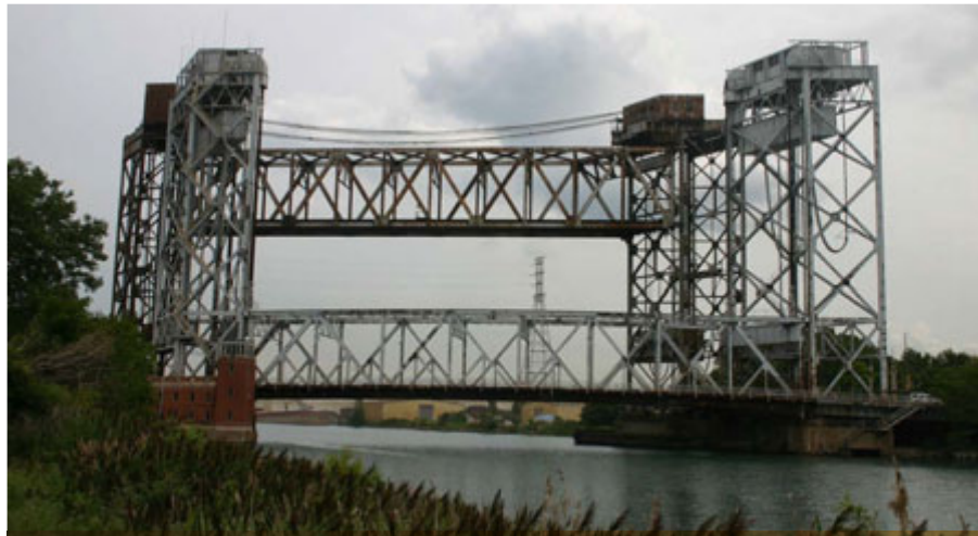
Existing Historic Torrence Bridge - Reconstruction beginning in 2012
