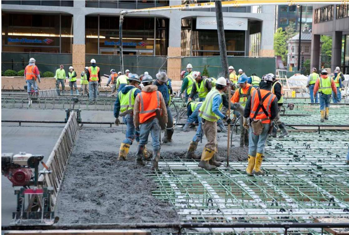
Where existing P.C.C. pavement exceeds the thickness listed in Table 4.3-1, the thickness of concrete used for restoration must match the existing conditions. The final surface of the finished concrete shall be performed according to [IDOT SSRBC Article 420.09\(e\)](#).
