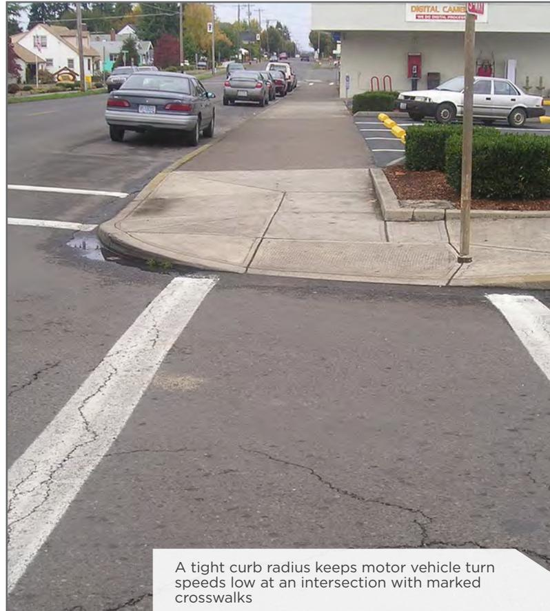
A tight curb radius keeps motor vehicle turn speeds low at an intersection with marked crosswalks
