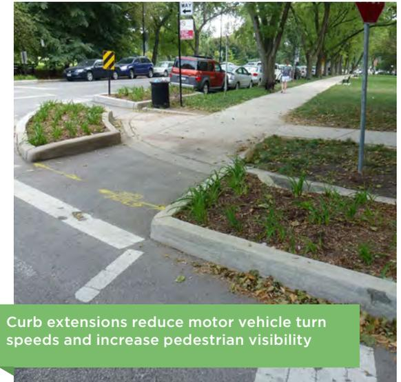
Curb extensions reduce motor vehicle turn speeds and increase pedestrian visibility
