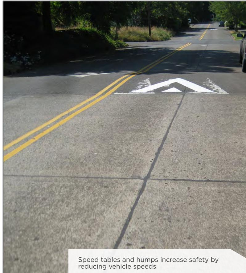
Speed tables and humps increase safety by reducing vehicle speeds
