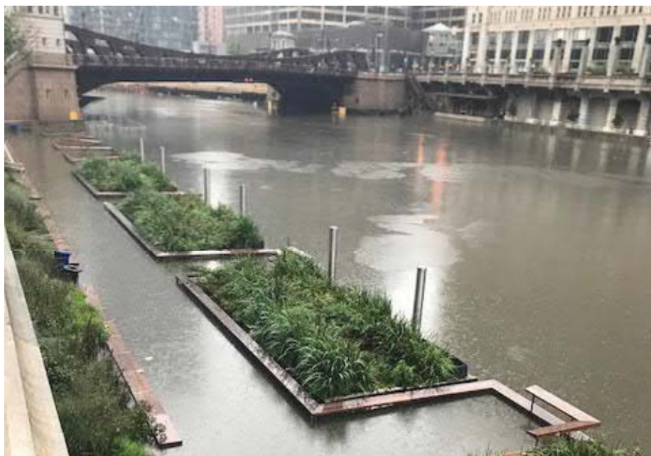
Figure 2-7: Main Branch Riverwalk between Franklin Street and Wells Street. The Main Branch Riverwalk was designed to permit temporary flooding during major storm events.
