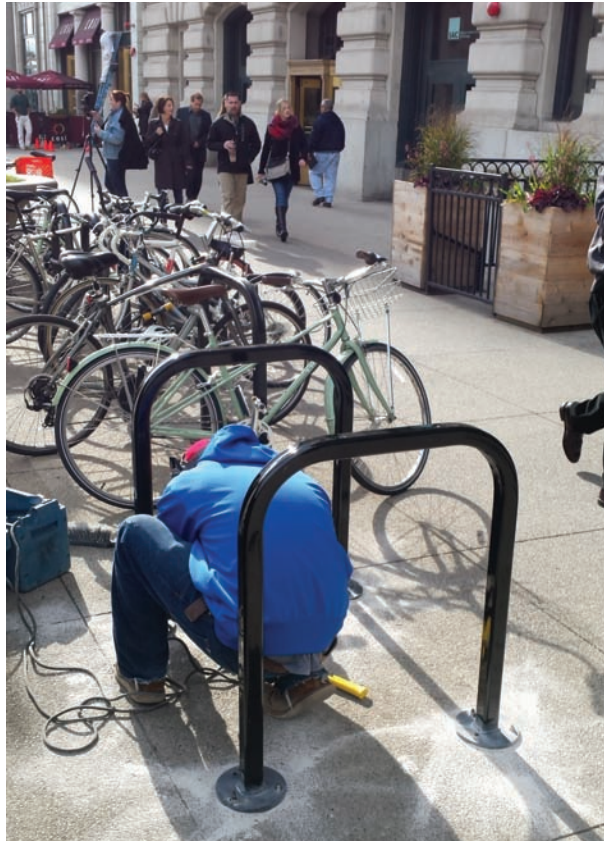
U-rack installation at 112 S. Michigan Avenue
