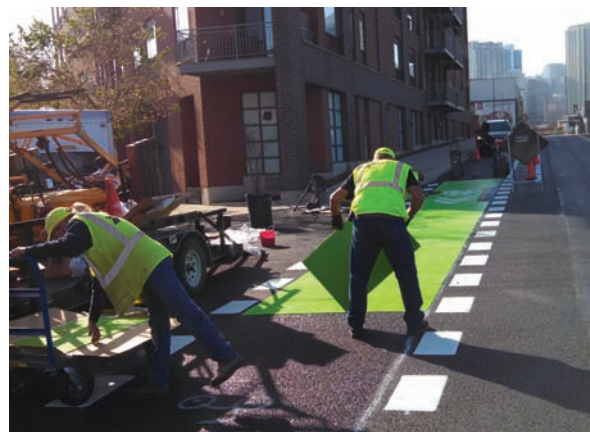
New striping and green pavement installation
