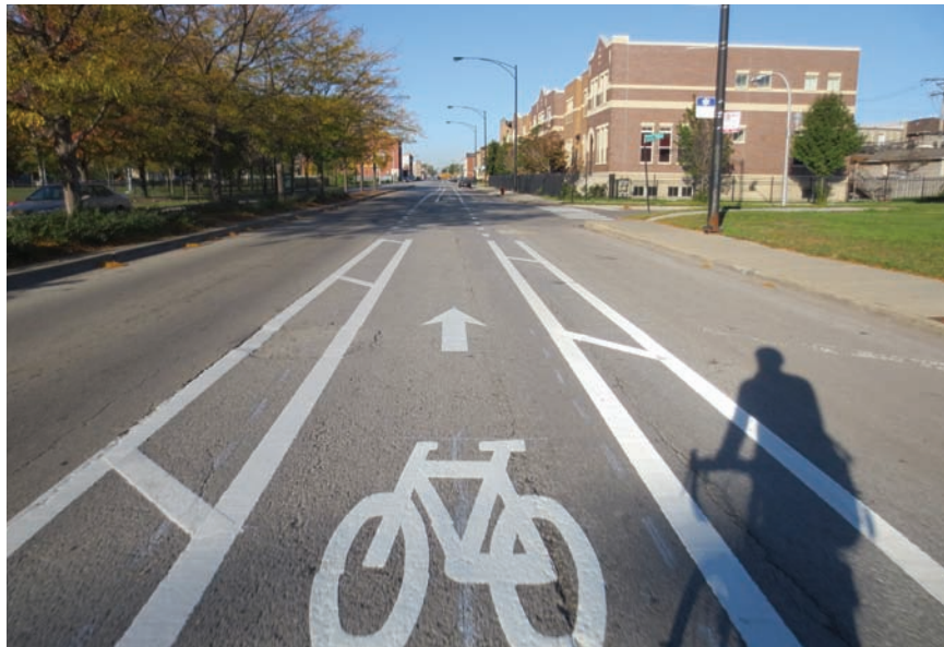
Pershing road diet and buffer-protected bike lane
