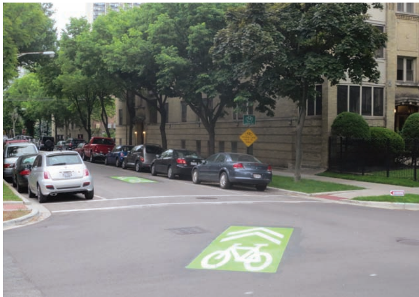
New pavement markings on Winthrop Avenue and Ardmore Avenue help to route bicyclists to the Lakefront Trail
