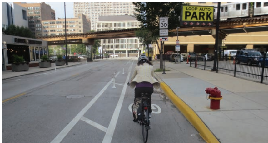
Barrier-protected lane on Harrison Street
