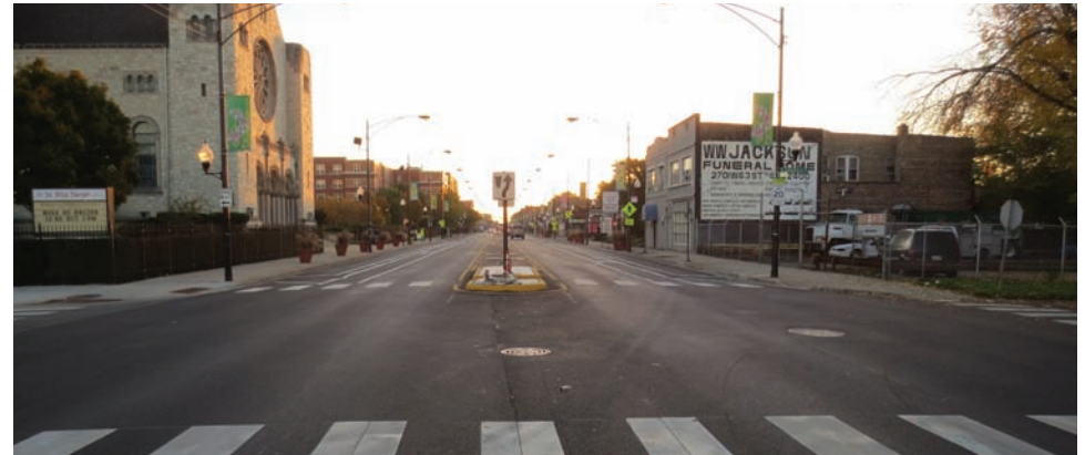
Pedestrian refuge island and buffer-protected bike lanes on 63rd Street road diet
