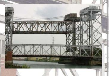
The Chicago Department of Transportation is rebuilding the historic Torrence Avenue bridge over the Calumet River. The vertical-lift bridge--the only city-owned bridge of its kind--was built in 1938. After more than seven decades, the aging structure requires a complete restoration.
