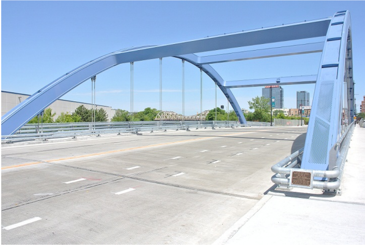
The newly constructed “tied-arch” bridge in the 1100 block of North Halsted Street.
