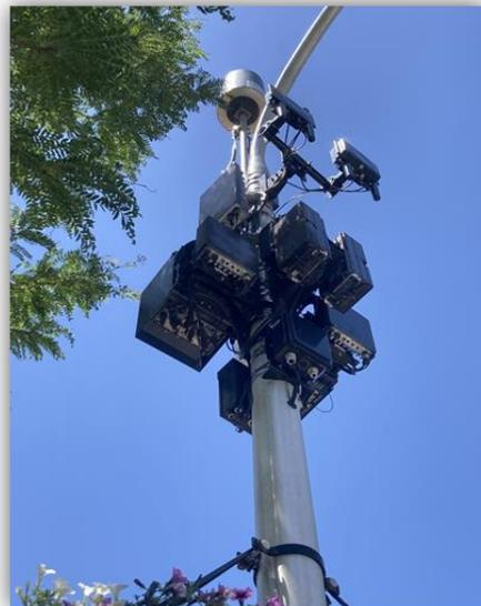
**Unshrouded non-concealed equipment, exceeding maximum volume and width, exposed wiring, and no consistent design uniformity**
