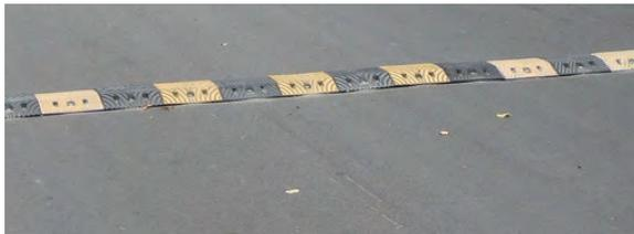
A speed bump is less than a foot in length and generally used in spot locations to reduce speeds.
