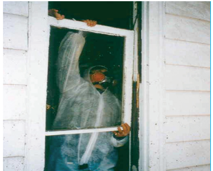
An abatement contractor removes a window identified with lead hazards
