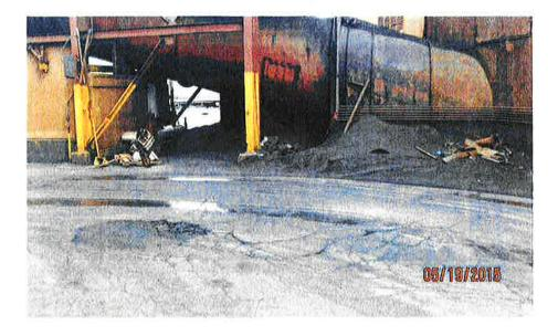
COMMENTS: Photo#9 Direction: SW Comments: Particulate dust accumulations around the silo feeding hopper and bucket elevator.
