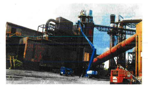
COMMENTS: Photo#6 Direction: NW Comments: Repair work on bucket elevator system, which transfer coke(petcoke and metcoke blend)into the silo.
