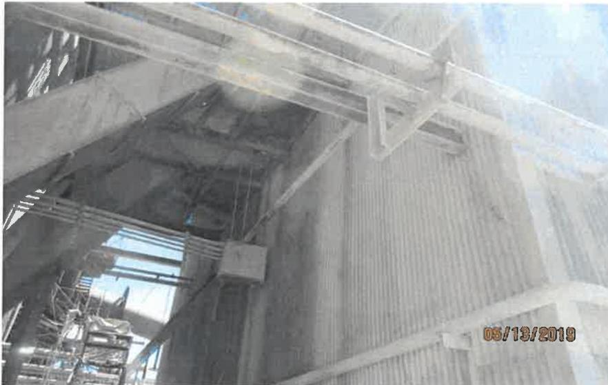
COMMENTS: Photo # 09 Direction: SE Comments: Emissions of particulate dust from openings on wall, door, pipes of BC # 3 (rail car loading station building) and BC # 10 building.
