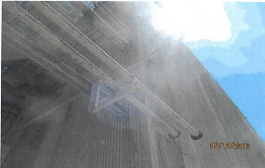
COMMENTS: Photo # 13 Direction: SE Comments: Emissions of particulate dust from openings on wall, door, pipes of BC # 3 (rail car loading station building) and BC # 10 building.
