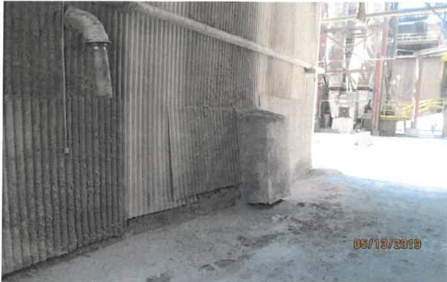
COMMENTS: Photo # 05 Direction: SW Comments: Accumulation of particulate dust on the ground, outside BC # 3 (rail car loading station building) & BC # 10. Also on walls, beams, pipes & other outside structures.
