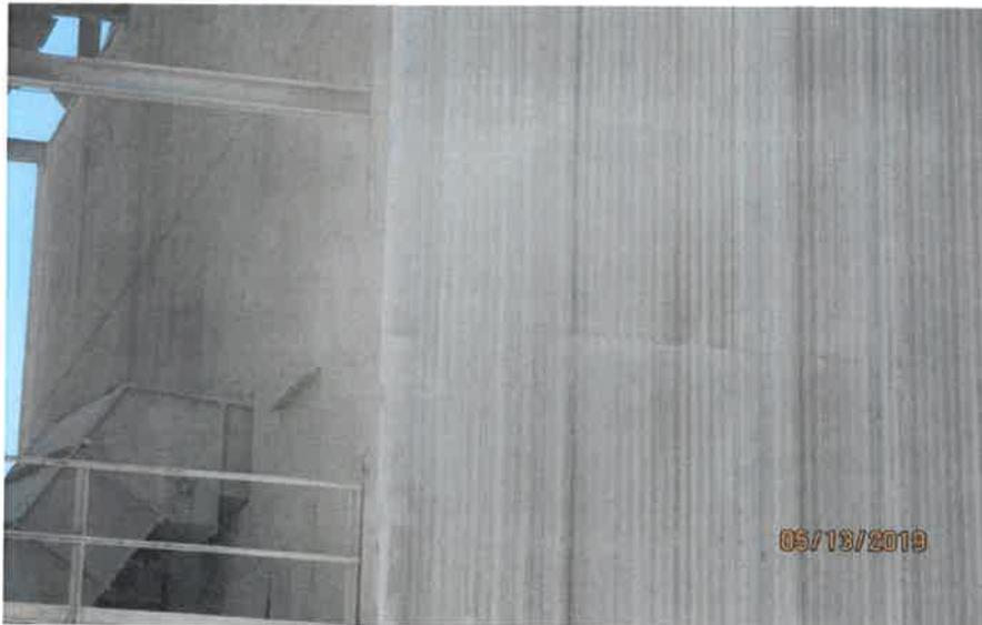
COMMENTS: Photo # 11 Direction: SE Comments: Emissions of particulate dust from openings on wall, door, pipes of BC # 3 (rail car loading station building) and BC # 10 building.
