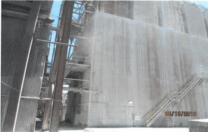
COMMENTS: Photo # 018 Direction: SE Comments: Emissions of particulate dust from openings on wall, door, pipes of BC # 3 (rail car loading station building) and BC # 10 building.
