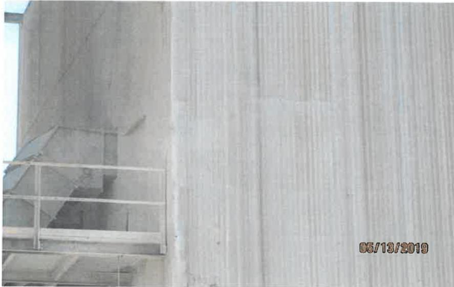
COMMENTS: Photo # 15 Direction: SE Comments: Emissions of particulate dust from openings on wall, door, pipes of BC # 3 (rail car loading station building) and BC # 10 building.
