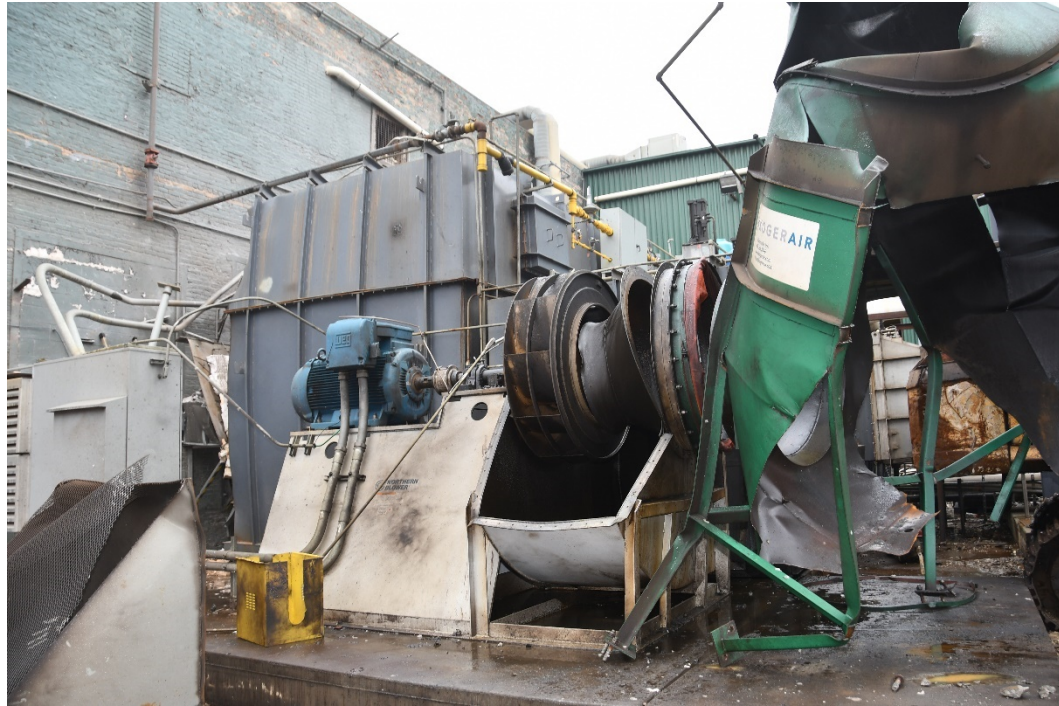
Figure 9. Photograph of the blower adjacent to the RTO. The green ducting on the right was the elbow of the ducting connecting the filter and the RTO. The fresh air damper is visible in the bottom left corner of the image.
