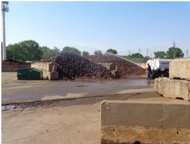
**Image 13:** Water truck applying water to Pig Iron pile prior to disturbing.
