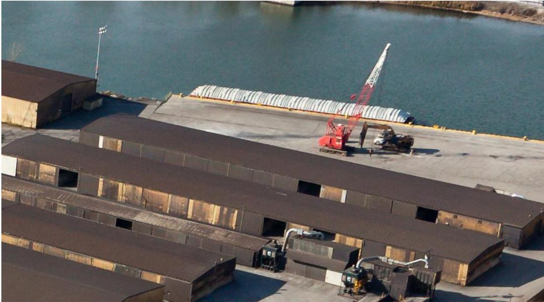
**Image 9:** Chicago Arrow Terminal dock area, single 200' barge covered with 9 stackable fiberglass lids. Note that all travel surfaces are paved.
