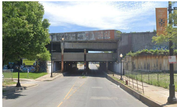
NEW METRA STATION AT 79TH ST
