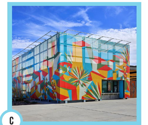
C FACADE INSTALLATION
