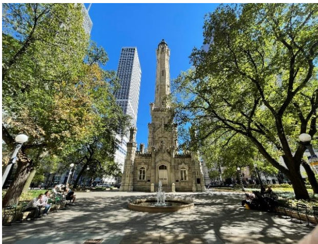
Water Tower and plaza, looking west.
