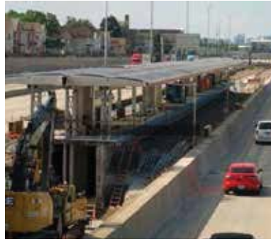
Red Line South Reconstruction
