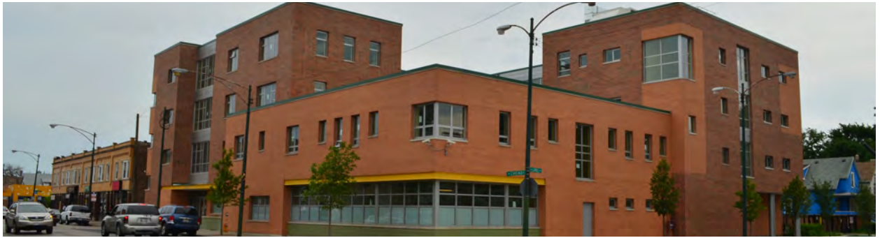
New Moms Facility at Chicago Ave and Loretta Ave
