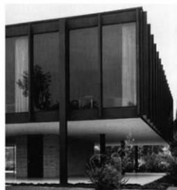
EXAMPLE: EXTERIOR METAL FINES AT WINDOW WALL
