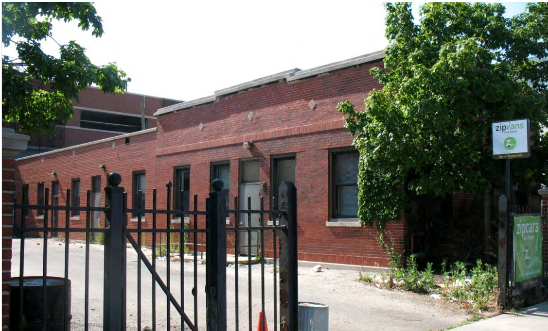
Top: The police station has a small auxiliary building, built circa 1931, that is located on the north side of the building. It originally was physically separate, but was connected to the police station by a narrow connector in 1994. Bottom: North of the police station is a one-story garage building built circa 1931. Neither of these small buildings are considered significant features for the purpose of this proposed landmark designation.
