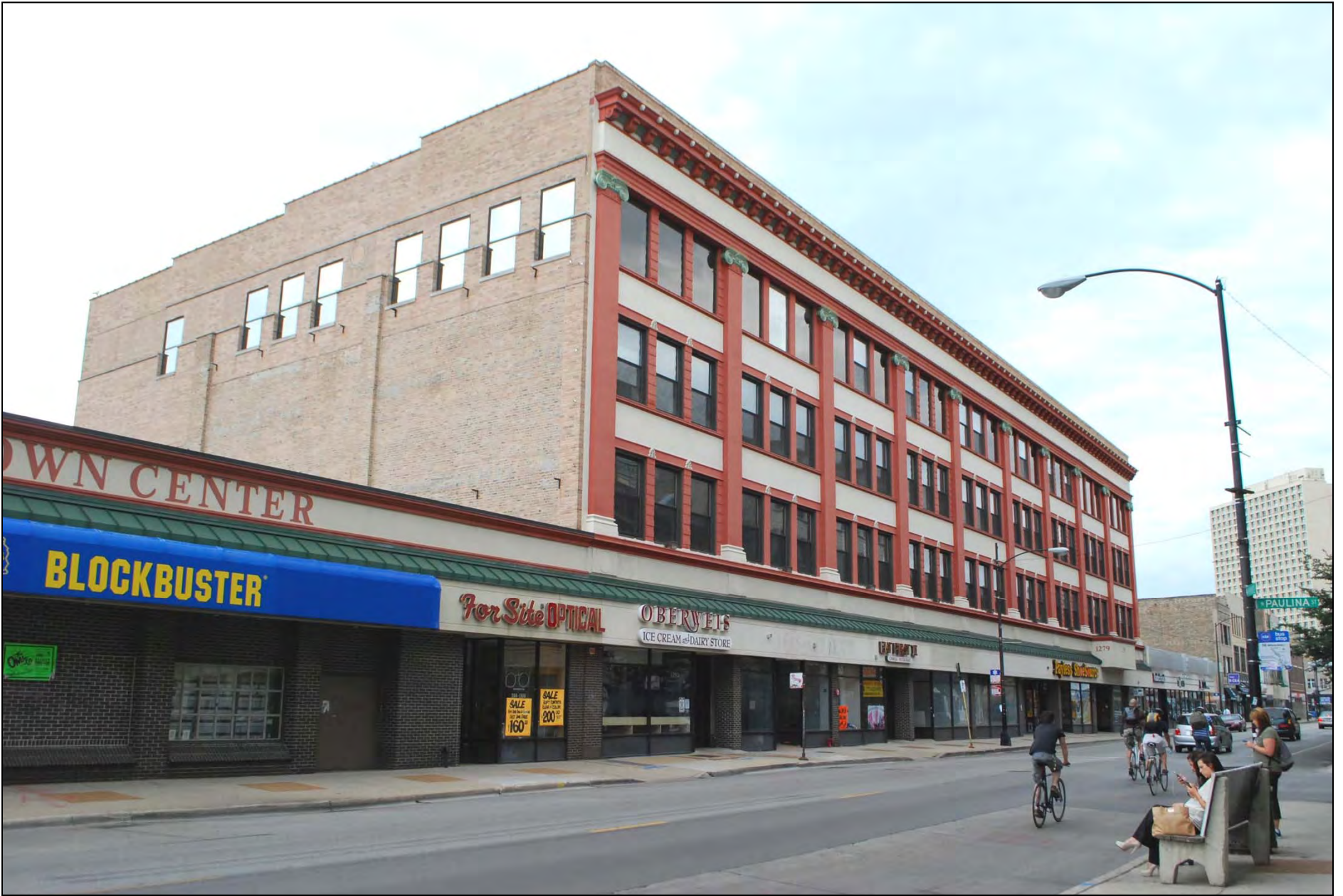
North and west (main) elevations, Looking south on Milwaukee Avenue (2012).
