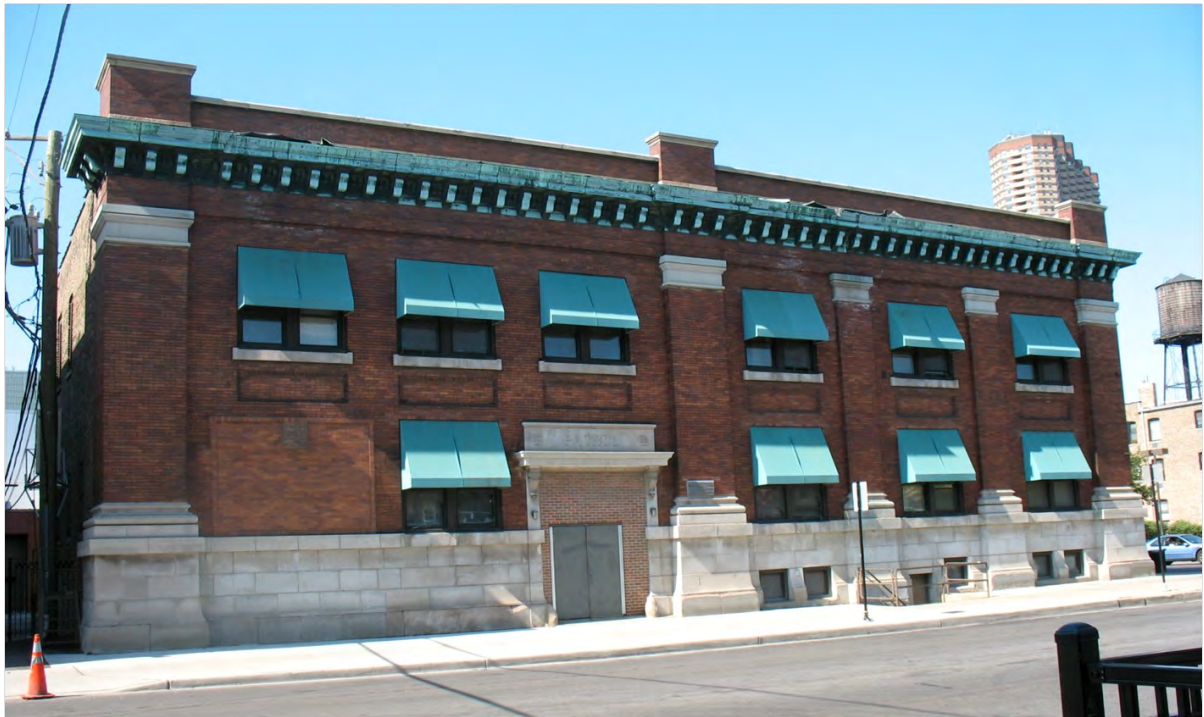
The 42nd Precinct / Town Hall Police Station is two-stories in height and built of brown brick and limestone trim. Top: A view of the building's Halsted Street façade. Bottom: The Addison Street façade.
