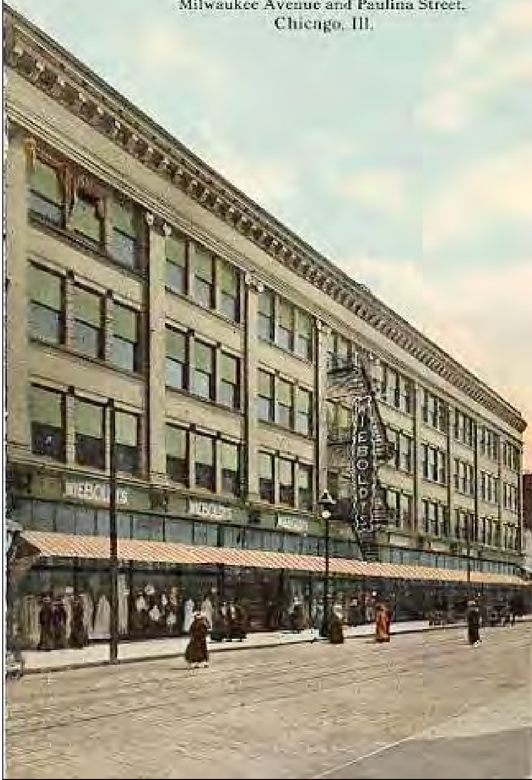
Image 3: West elevation circa 1915 showing completed elevation.
