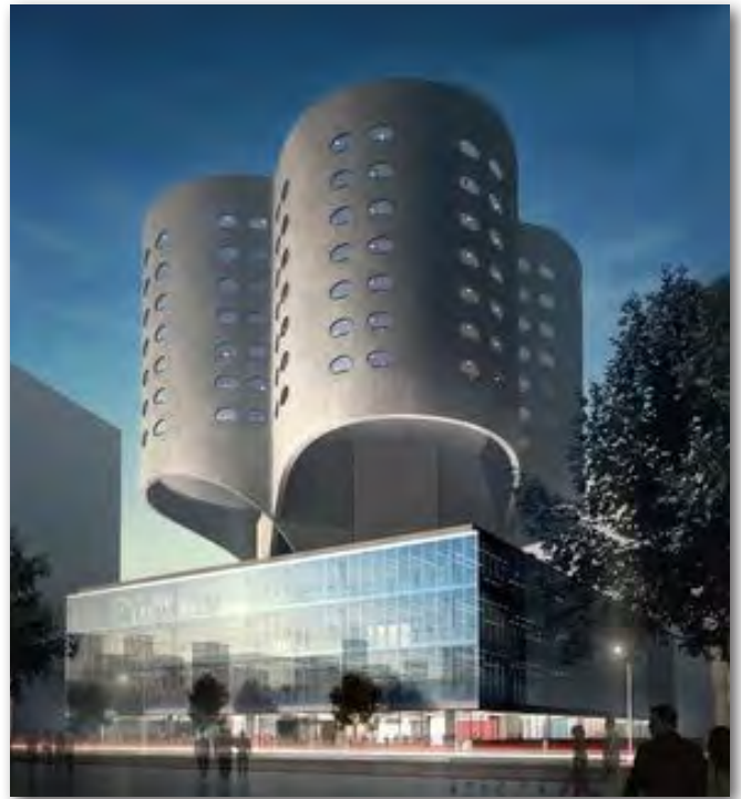
A rendering of Prentice Hospital depicting how it would look following renovation, including replacement of existing glass curtain wall and removal of non-original fifth floor addition to the base. (Source: Landmarks Illinois’ reuse study)
