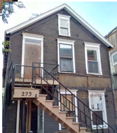
after siding removed
