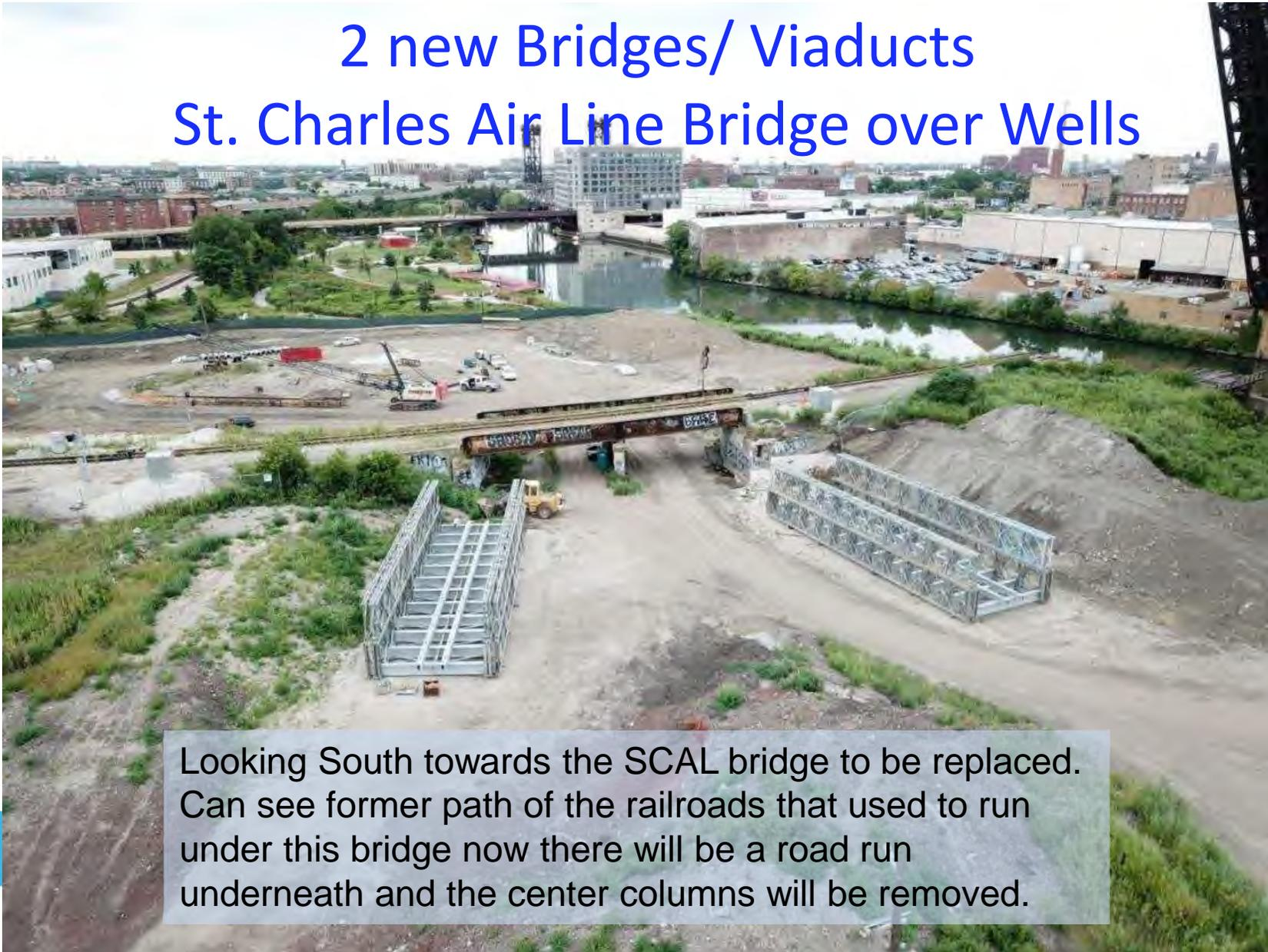
Looking South towards the SCAL bridge to be replaced. Can see former path of the railroads that used to run under this bridge now there will be a road run underneath and the center columns will be removed.
