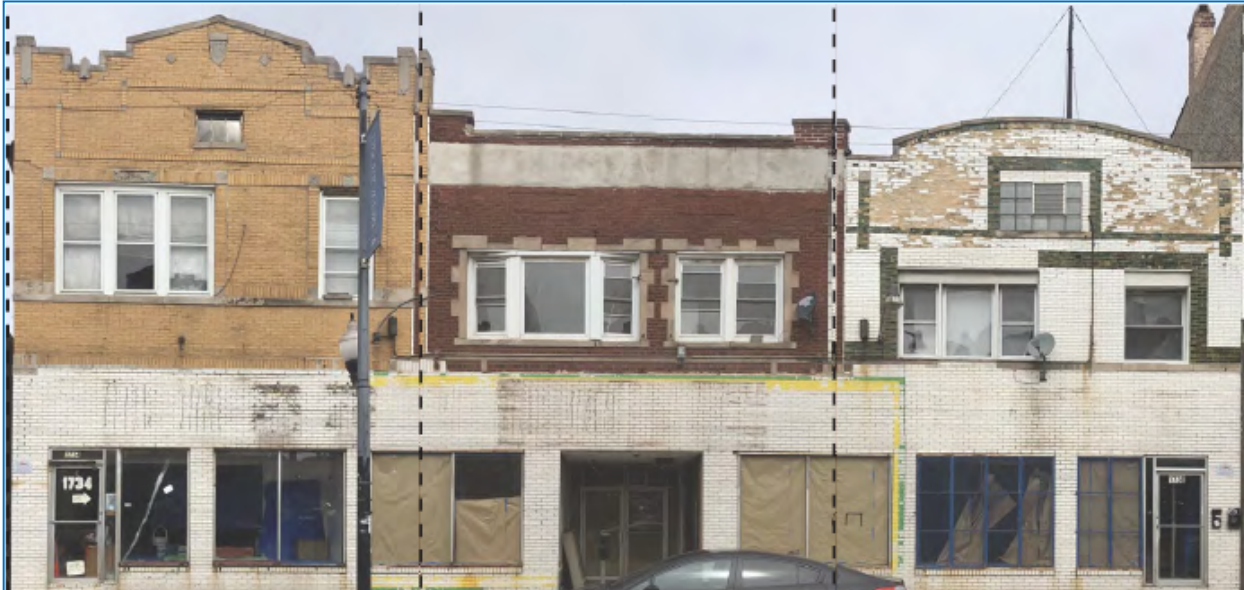
1730, 1732, 1734 W. 18 th Demolition application denied due to landmark district. Buildings being rehabbed.
