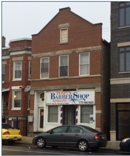
2038 W. 18 th Demolition application denied due to landmark district.
