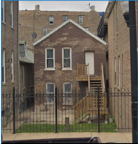
1822 S. Throop Demolition approved building deemed “Dangerous & Hazardous”
