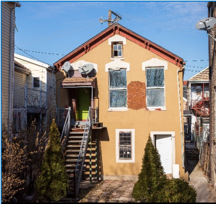
1330 W. Cullerton Demolition application denied due to landmark district.
