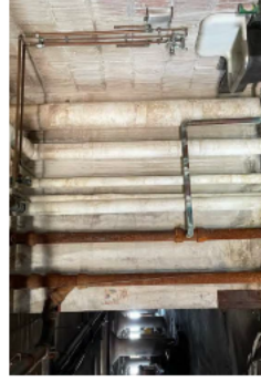
H - Existing piping and plumbing fixtures
