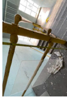
H - Guardrail at Stair C
