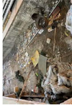
B - Rubbish at loading dock
