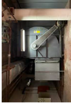
C - Abandoned mechanical units
