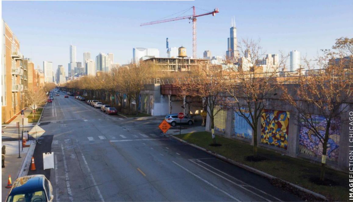
Existing Condition along Hubbard Street
