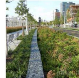
2 Enlarged landscape parkway with stormwater infiltration and mitigation features
