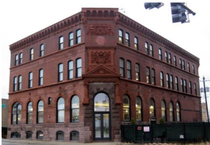
Schoenhofen Brewery 1886 18th St. and Canalport
