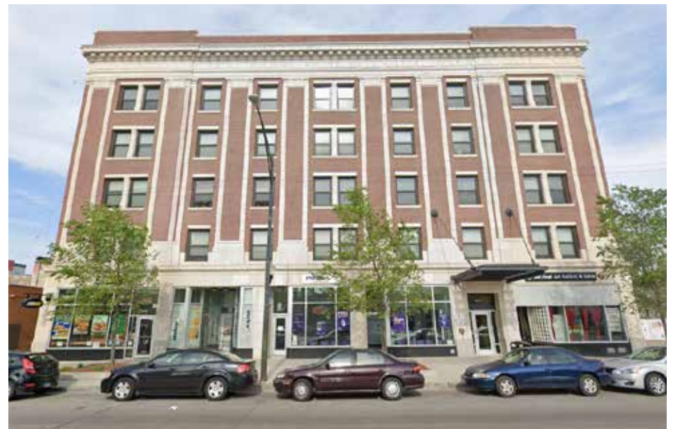
The Strand Residences, a renovated historic building on Cottage Grove Avenue
