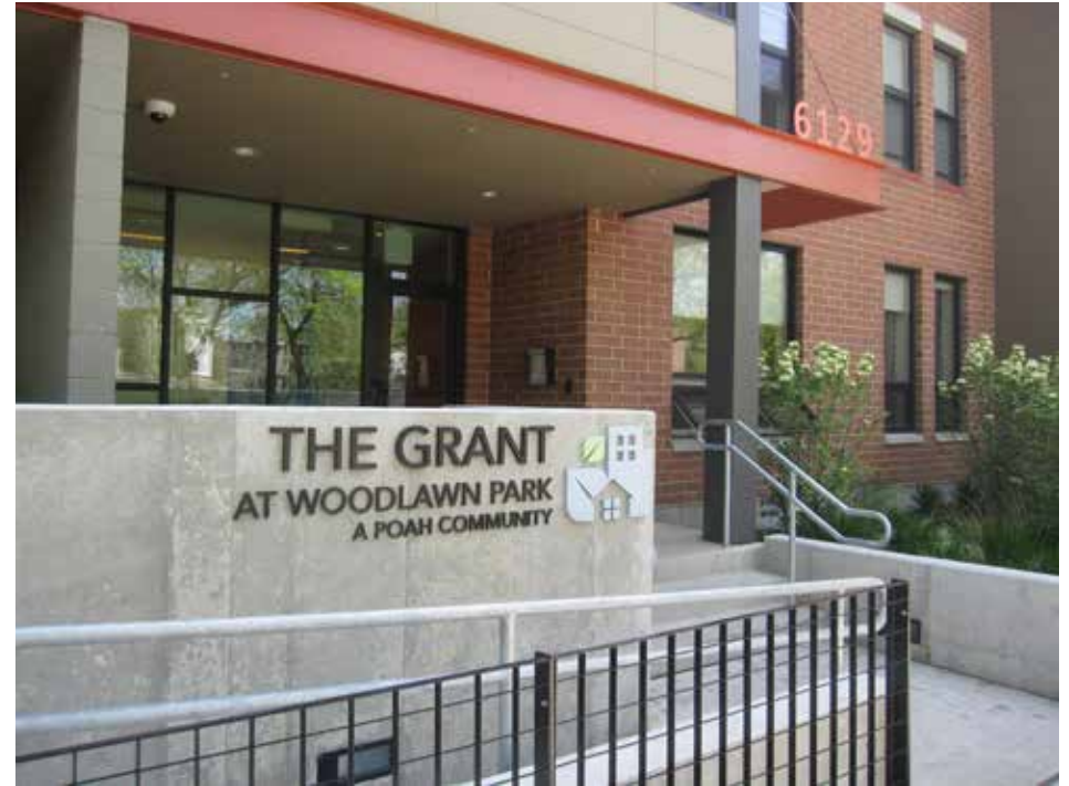
The Grant, a POAH development along Cottage Grove, opened in 2013
