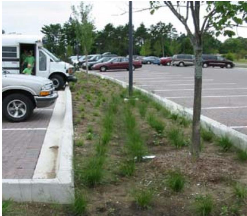
**Figure 3.8 Example of Bioswale and Permeable Pavements**
