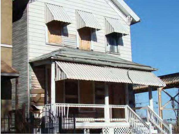
The porch roof on 5924 La Salle is deteriorated and the shingles have become dislodged.
