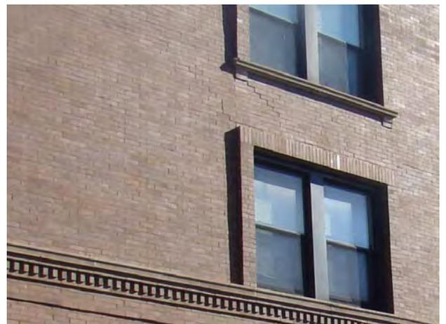
Step cracking in the bricks on 108/110 58th Street.
