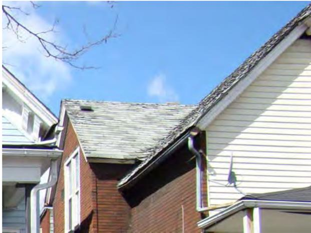
Deteriorated shingles on 5530 La Salle Street.
