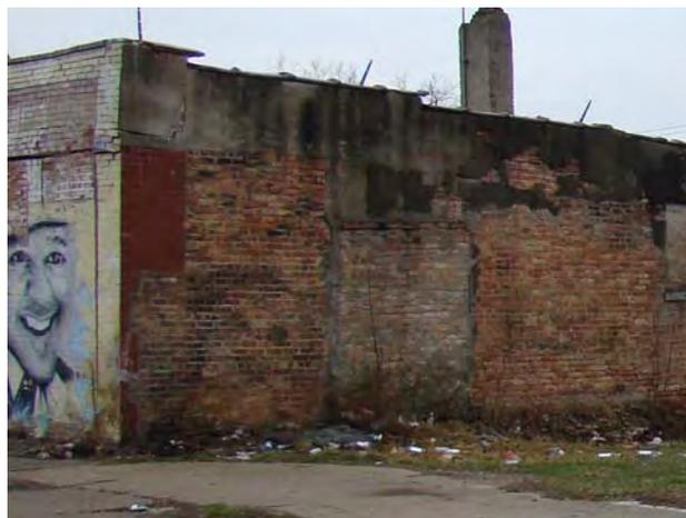
The rear wall of the previous commercial building is sagging and bricks have fallen out of the wall.
