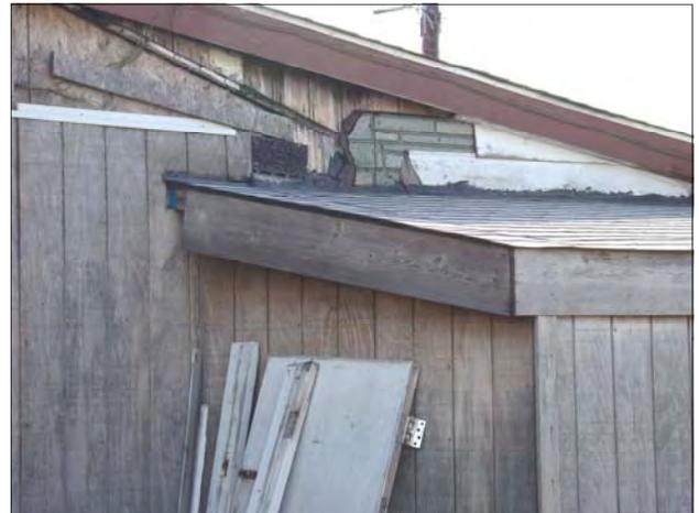
An example of deteriorated building components (roofing material, siding and fascia, etc.) documented in the Area.
