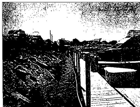
Recent improvements to docks draw contrast with the waste concrete used on the shoreline for bank stabilization.
