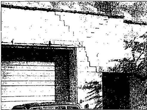
Evidence of major structural damage to a load-bearing wall (dilapidation).
