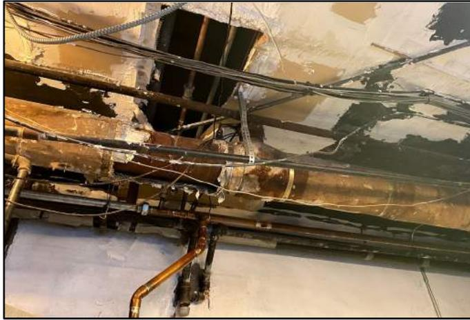
Asbestos containing AirCell pipe wrapping in boiler room
