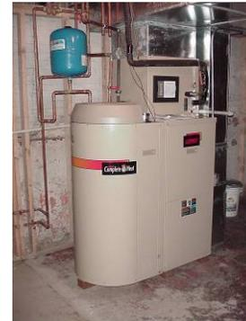
Combination systems merge domestic hot water and space heating into a single appliance. Water is heated within the unit and piped through an air handler to supply space heating through a standard duct system. Commonly available systems are high-efficiency, sealed combustion units. An air conditioning coil can also be included.
