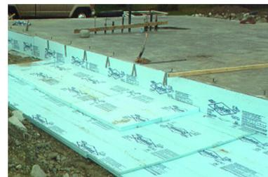
Typical foundations are installed below the frost line to prevent “frost heaving”. A FPSF uses insulation to raise the frost line just below grade allowing foundations as shallow as 12 inches. Insulation installed horizontally from the foundation is used to keep the soil warm. Good site drainage is also required to keep water from soaking in and around the foundation.
