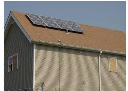
The PV system may be connected to the utility grid. This means that batteries are not required. Whatever extra solar electricity is generated is fed back to the utility, and any extra needed by the occupants is drawn from the utility as in a typical house. This credit applies only to solar electric systems. For active solar space heating see feature 220.2, and for solar domestic water heating see feature 230.1.
