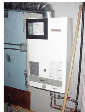
“Tankless” water heaters eliminate the tank and associated standby losses. Water is heated as it is needed. Consequently, tankless heaters can offer significant improvements in efficiency and performance.
