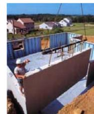
insulation already installed and furring strips pre-attached to the stud face to further simplify site construction. Panels range in size from 2 to 12 feet in width and 8 to 12 feet in height. They are typically installed by a crane, which lifts the panels into place on top of 4-6 inches of compacted stone. The stone facilitates sub-slab drainage and transfers the load from the foundation wall.
