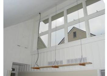
A clerestory is a high wall with a band of glazing along the very top. The clerestory wall usually rises above adjoining roofs allowing both daylight and sunlight into the space. Operable clerestory windows and/or operable skylights are commonly used to provide natural or passive stack ventilation.
