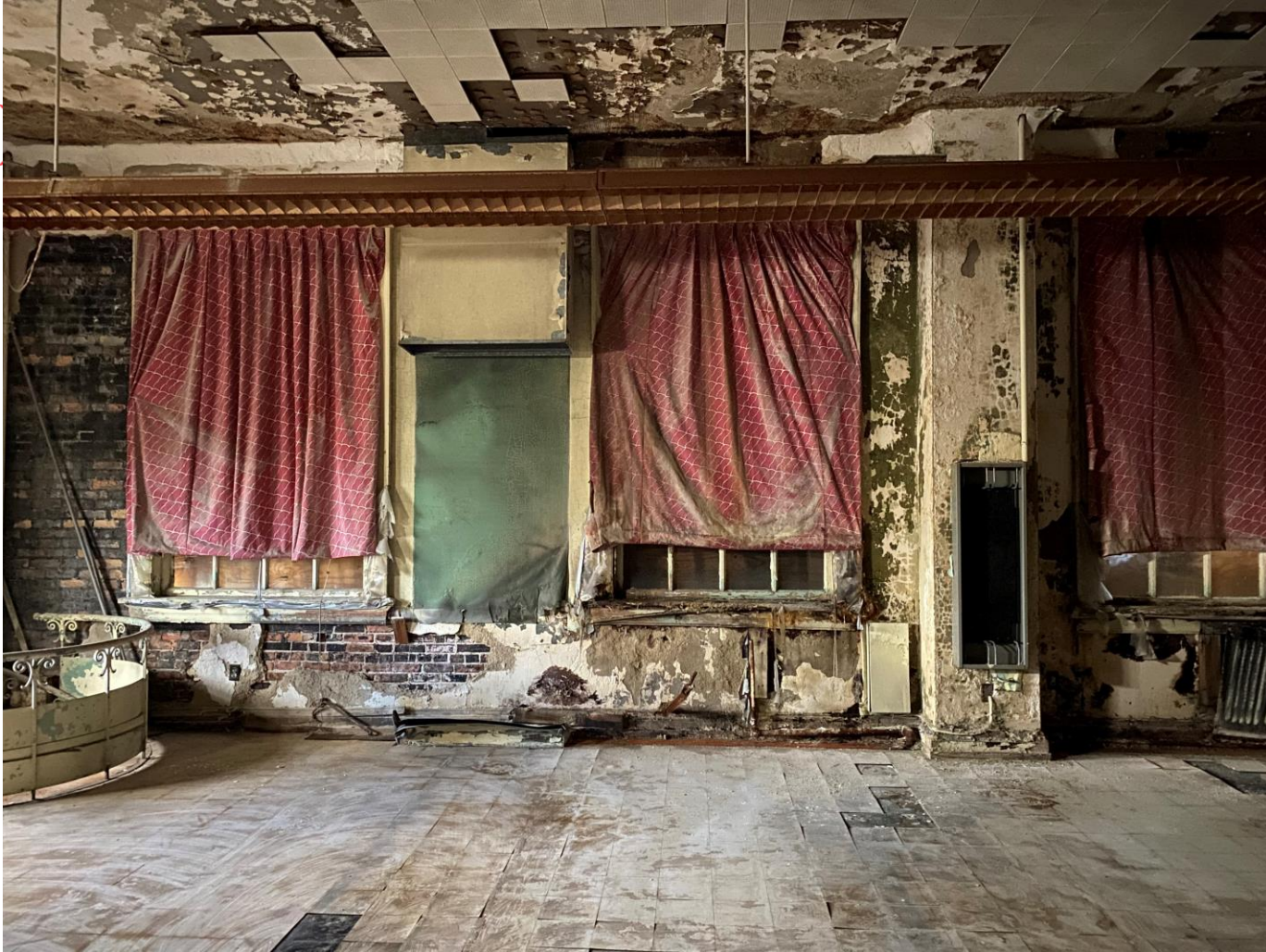
Second Floor abatement needed for floor and ceiling tiles Plaster crumbling from walls and ceiling trim.
