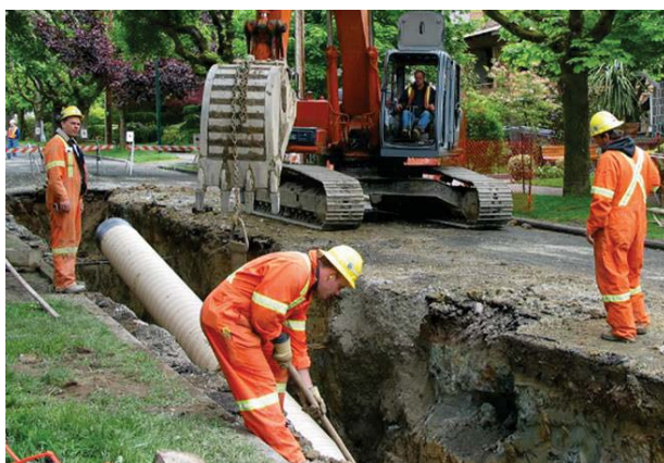
Figure 20: Excavation of Sewer Lines
