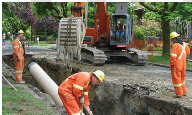
Figure 20: Excavation of Sewer Lines
