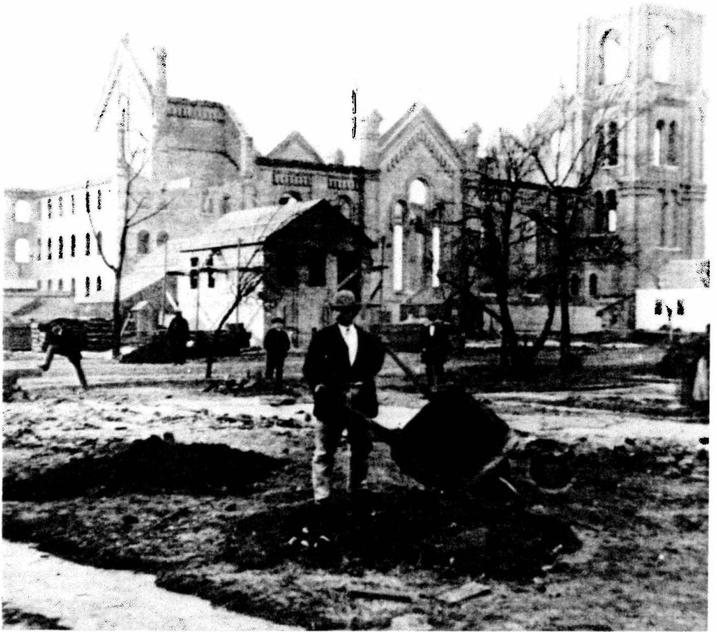
This photograph, taken shortly after the Chicago Fire of 1871, shows the ruins of St. Michael's Church. The double walls on the south, east, and west ends of the church withstood the fire. Within one year and three days after the fire, the industrious parishioners of St. Michael's Church rebuilt the damaged structure. Chicago cottages like the one pictured in the center of the photograph dotted the area within days after the fire and were sometimes referred to as "relief shanties."
