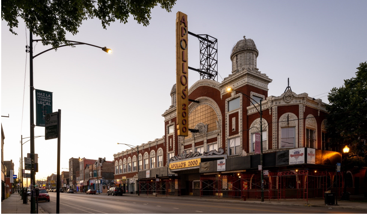
A current photograph of the main elevation facing Cermak Road. The theater entrance is marked by a large arch flanked by towers topped with domes. The cream colored terra cotta was manufactured by the Midland Terra Cotta Company of Chicago.
