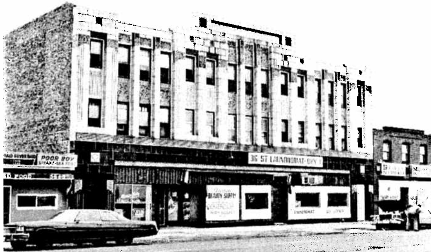
The street facade of the Chicago Bee Building, shown here in a 1985 photograph, is a colorful essay in Art Deco terra cotta. The ground story is clad in black with gold trim, and the upper two floors in shades of green.
