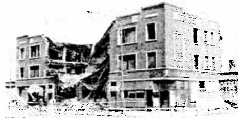
The Jordan Building was demolished in 1985, after it collapsed following years of brick thefts from a loadbearing rear wall.
