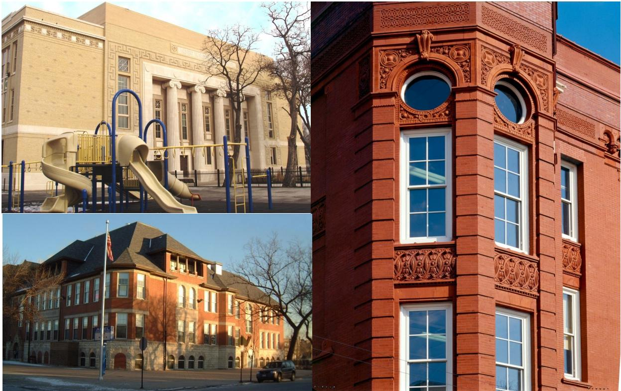
**Exterior Wall Materials:** Load-bearing brick masonry in a variety of colors, with limestone (limited use of sandstone), and/or terra cotta detailing. Pressed metal cornices were common.
