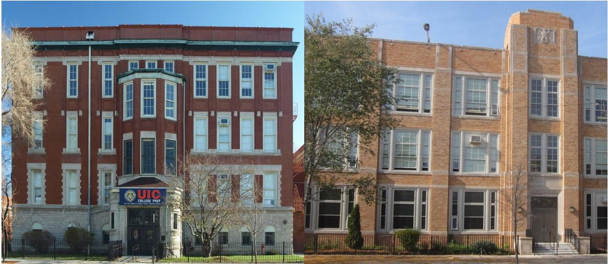
**Fenestration:** Punched window openings. Earlier buildings had brick arch or stone lintels; later buildings used steel lintels that allowed for wider openings. Classroom windows were wood-framed double-hung, sometimes with a fixed transom. Windows at stair towers or specialty spaces were sometimes arched or round. In most cases the original windows have been replaced with aluminum-framed windows of similar configuration.
