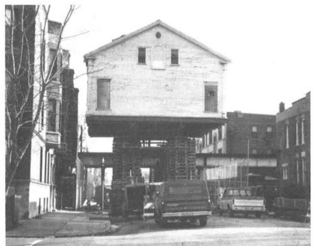
after midnight on Sunday, December 4, 1977, when El traffic was at a minimum, all train service on the line was halted. Temporary rails were laid across the tracks, cables were attached to the house, and trucks on the street below pulled the house slowly across the tracks. Despite the very cold weather, about 2,000 people gathered to watch as the house moved over the tracks and onto another set of cribs on the east side of the El. Soon the trains were running past the house once more.
